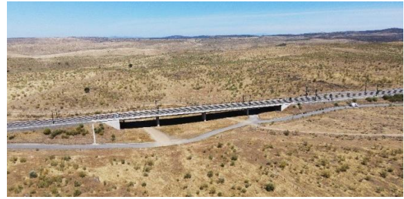
Figure 2. Drone view of the viaduct.
