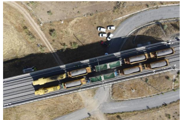
Figure 3. La Plata viaduct during the execution of a static load test.
